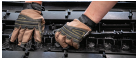
Step 2. Press clips together to interlock tiles and then secure tiles to surface
