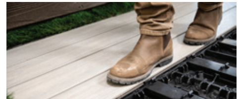
Step 3. Step down to snap boards in
